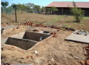
Building the tops for our septic system
