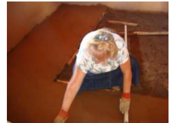
Jaynie, working on our special floors of cow dung, clay and sand.
