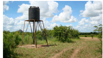
The 5,000 liter water tower is in place.
